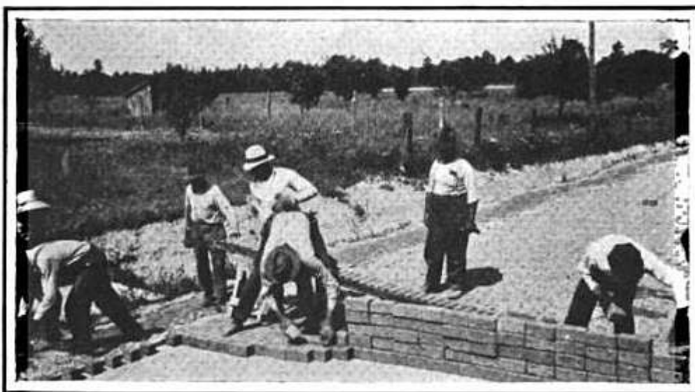
BRICK-ROAD CONSTRUCTION
